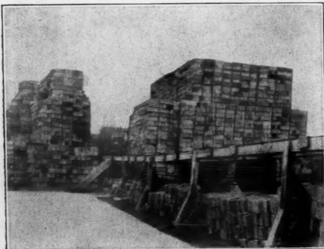
Storage for tile. Note cable conveyor with steam pipes below for curing
